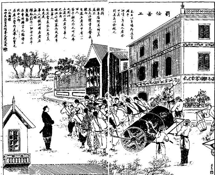
figure 42 Street repairs: precursor of the steamroller
